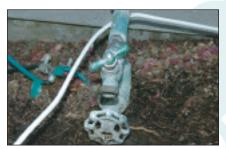
Your shutoff valve, which is usually located below a faucet at the front of your home, is the only location residents should turn off water. Check your water main yearly by turning it on and off. If you don't have a shutoff valve, consider having a plumber install one.
